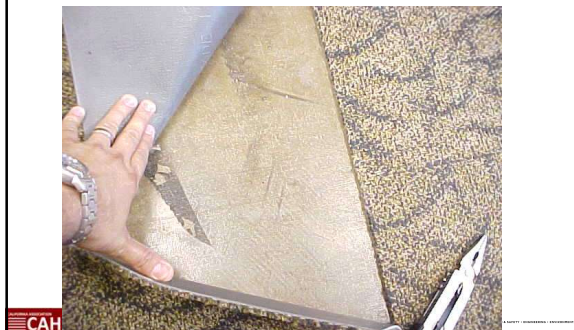
Example of an acceptable area under glue applied carpet squares
