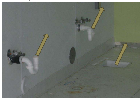
Vacant Suite or TI (Dry Trap), No Sinks (Unhindered Sewer Gas Pathway)
