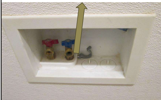
Unused Washing Machine Drain
