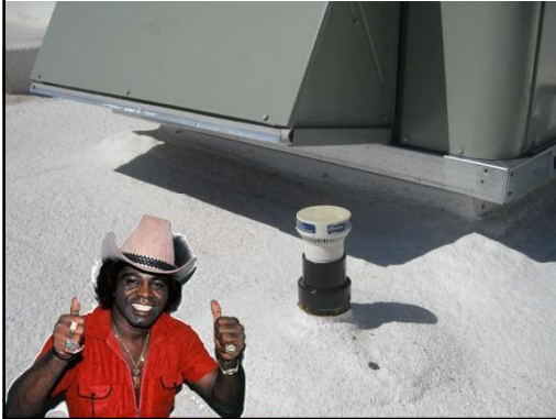
Sewer Gas, Vent too close to OA
