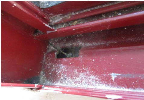
Penetration Points Window Sills, Door Tracks, Gable Vents, Etc.
